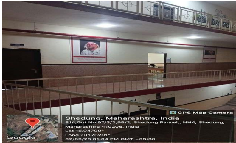
LED Lights in Corridor
