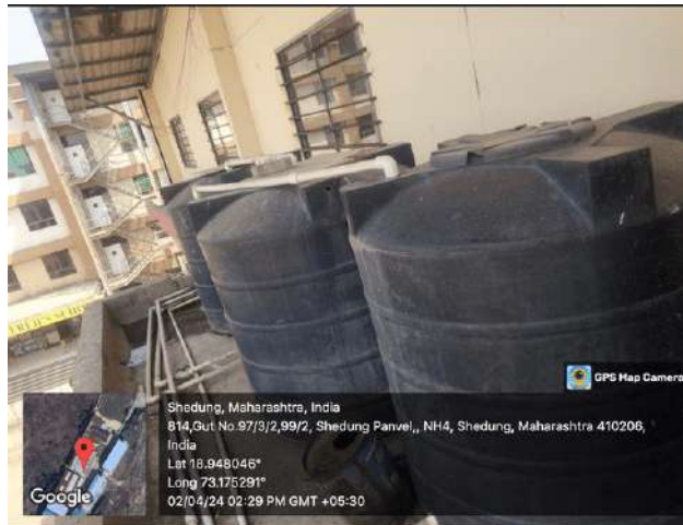
Overhead Water Tank
